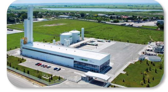
2017-2019 New SIAD Production Facility – Hungary Contract Value: €26 million Engineering and Health & Safety Planning and Construction Supervision
